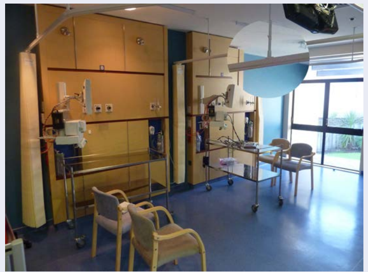
After adaptatrack is installed
